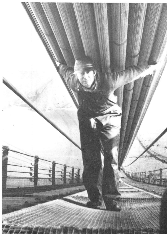
The Center directed the official history project for the 50th anniversary celebration of the building of the Golden Gate Bridge. Photographs, oral histories, hard hats, and other material came to the Center during the spring of 1987 including a scrapbook on Fred Dummatzen who was one of the workers to die in the accident in February 1937. Here he is clowning on the Bridge for his buddies with the Marin headlands in the background. Courtesy Labor Archives and Research Center, San Francisco State University
